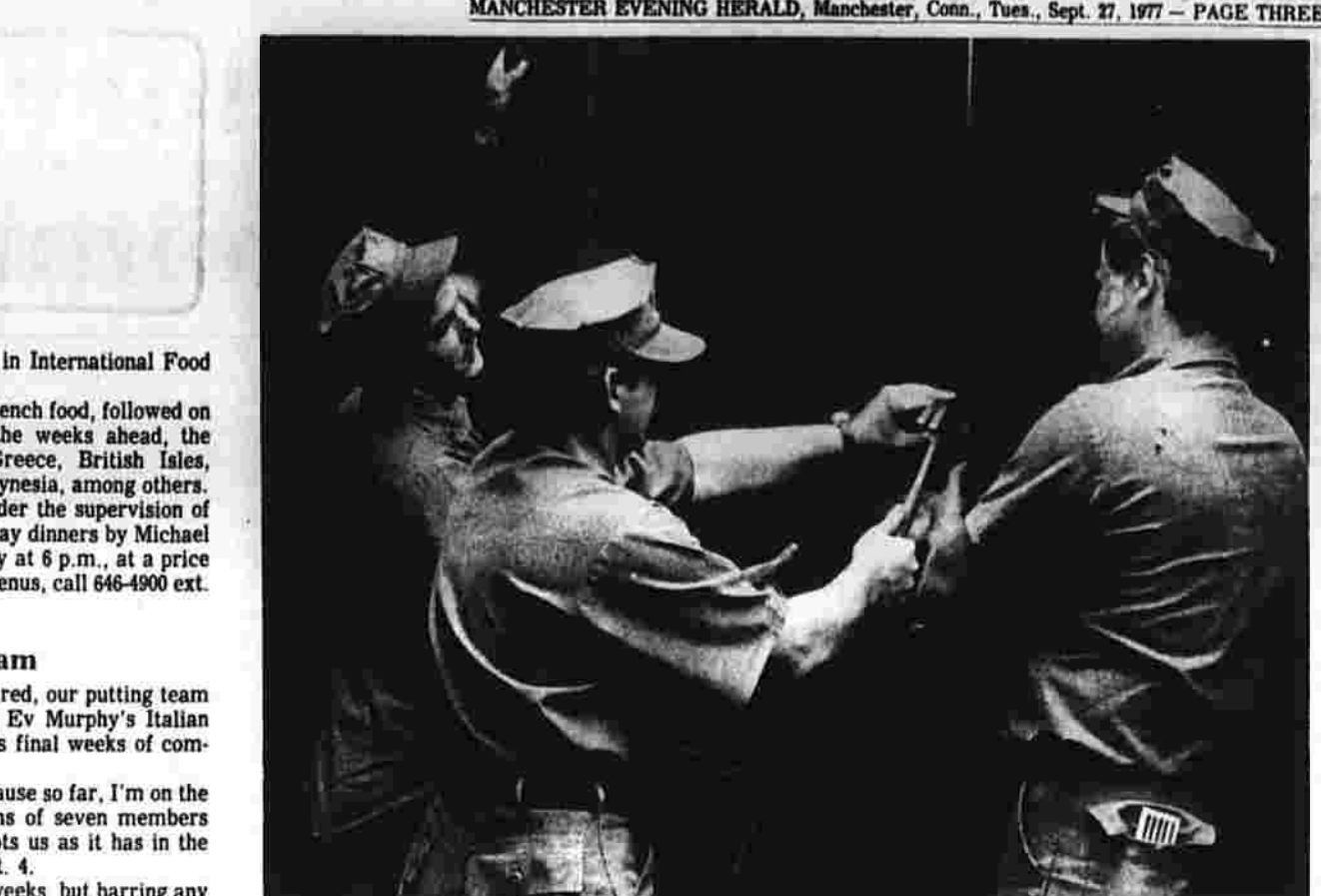
Lending a hand to repair buildings at Camp Johnson in Bolton, are U.S. Naval Seabee members, from left, Dave Lazzari, Chuck Barrera, and Terry Terricciano. Seabees instructed area Boy Scouts in maintenance procedures during repair session. (John Moffat photo)
